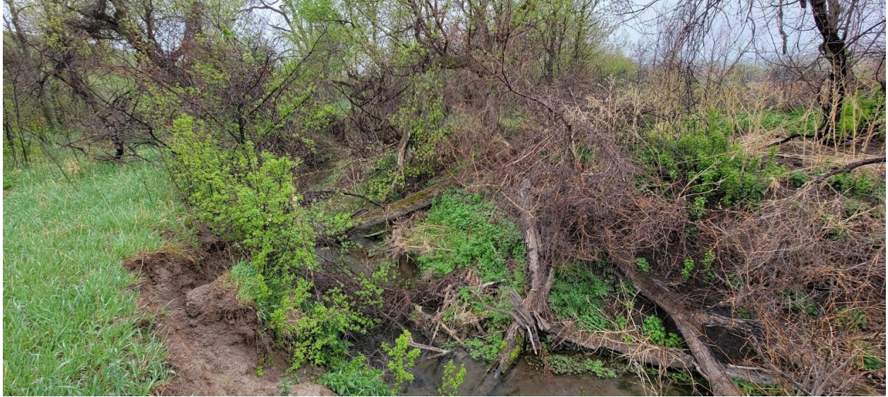
Figure 3-Preconstruction view of Bordeaux Creek WMA. Banks are full of woody debris and highly incised.
