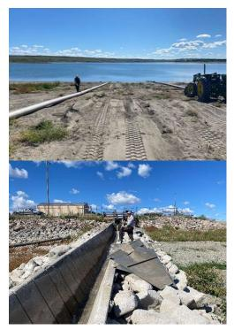
Placing the different sections of irrigation pipes and bolting the section together and pushing the whole works into the lake. The pumps sit on the bottom of the reservoir and push thousands of gallons of water per minute through the spawning station. That's me on the left checking 400ft of cable for abrasions or cuts that could short out the pumps.
