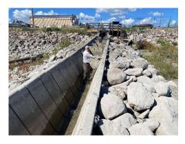
Here is the ladder after we started up the pumps and are pushing a little water. When both pumps are running full speed, about twice as much water will be running down the ladder than what is currently seen.
