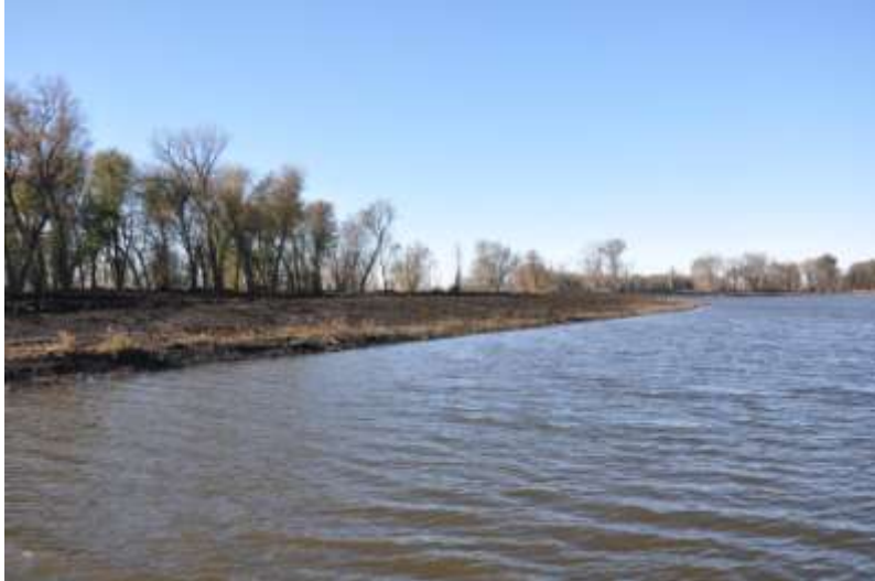
Figure 1. Photo of the tree clearing and berm in the Huron Island project area
