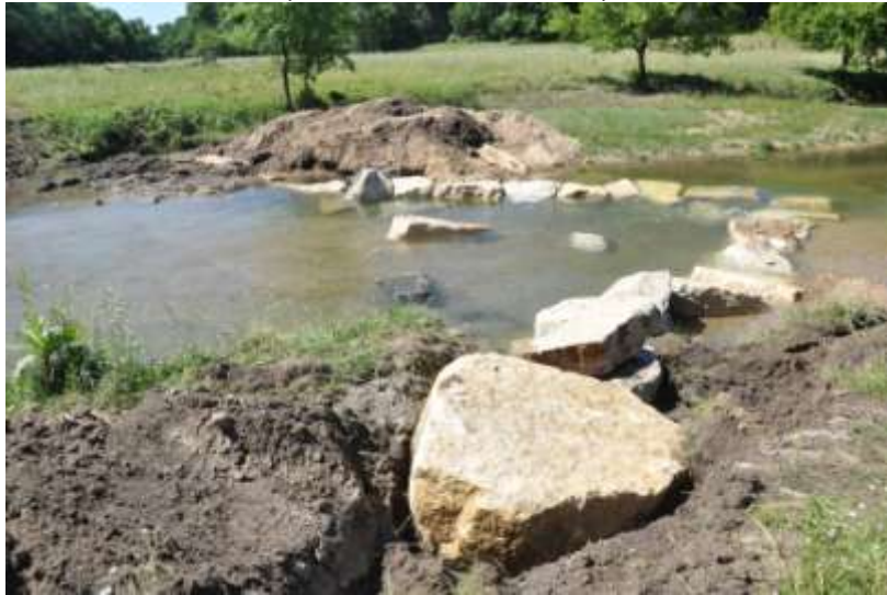
Figure 1. Upper Maquoketa River Habitat Project June 2016- Rock Weir
