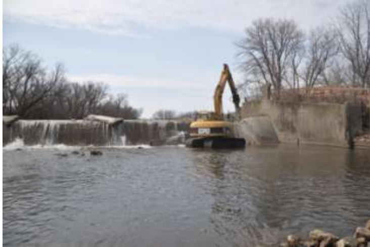
Figure 2. Buffalo Creek Dam Removal Project 2016
