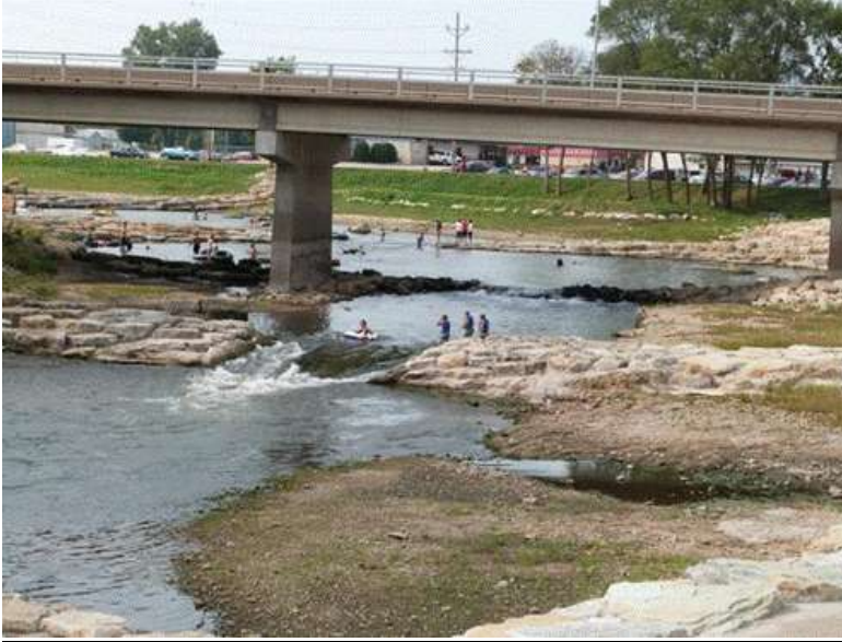
Figure 2. Manchester Dam following Whitewater Park construction
