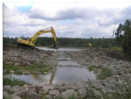
The newly created channel.
