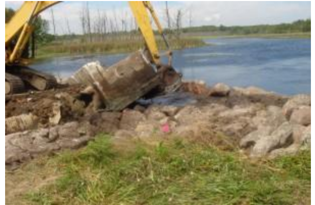
Removal of inlet structure at Pigeon Lake Impoundment
